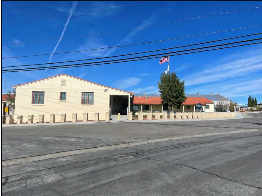
Photograph 5. View of southeast façade of the Training Center and court, facing northwest.
