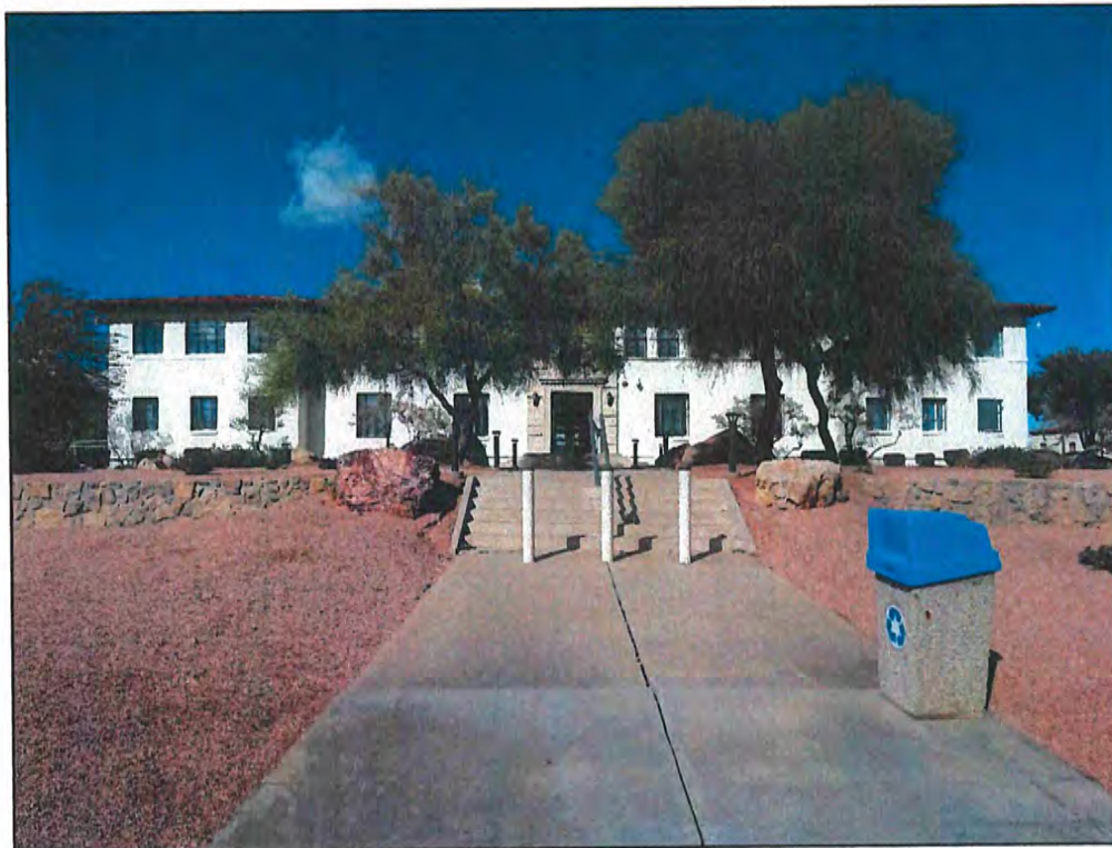
Figure A.4. View of Administration Building and Government Hill from concrete landing on central walkway, facing north.
