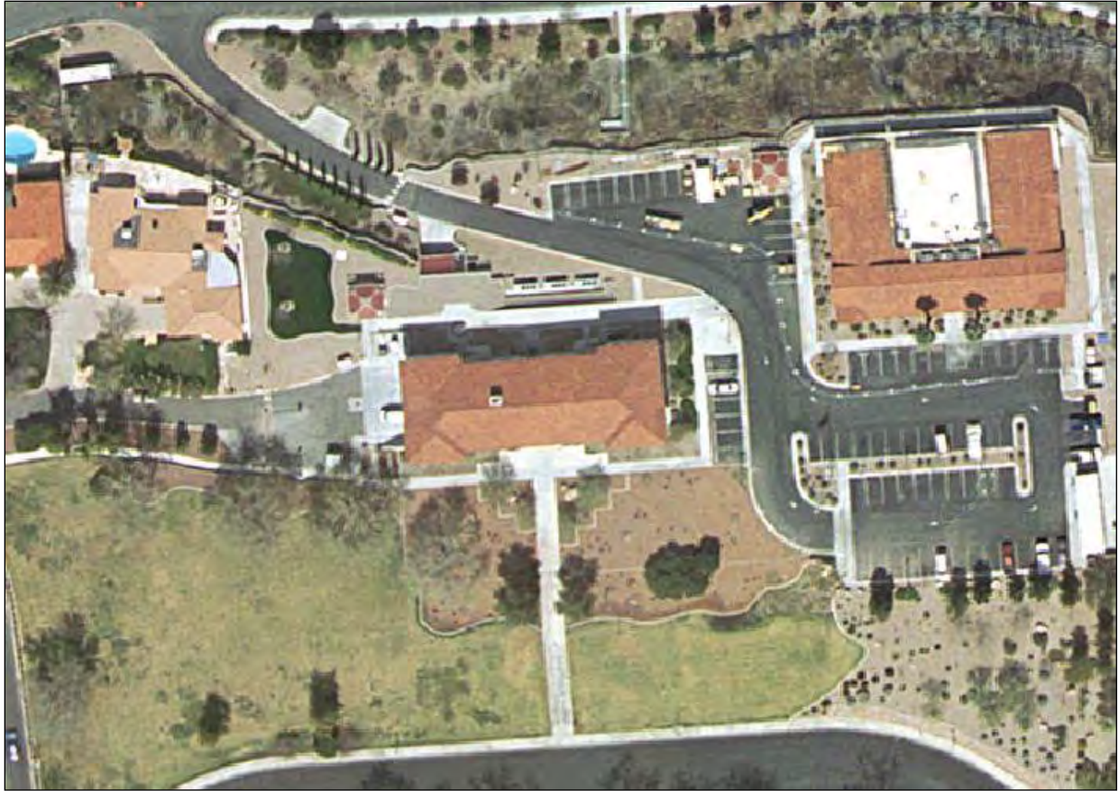
Figure 7. Aerial photograph showing the landscaping surrounding the Admin Building as it appeared in 2006 (Image courtesy of the Clark County Assessor, Las Vegas).
