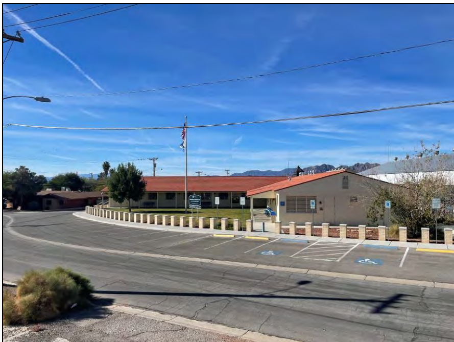
Photograph 8. View of Training Center and court, facing southwest.
