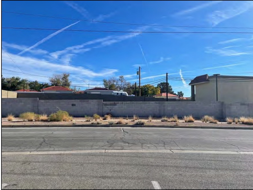
Photograph 11. View of north parking lot of Best Western Motel, directly across from Training Center, facing east.
