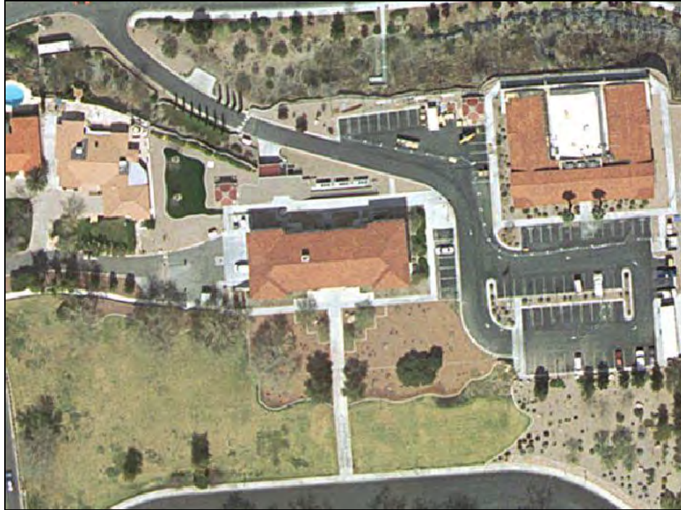
Figure 7. Aerial photograph showing the landscaping surrounding the Administration Building as it appeared in 2006 (Image courtesy of the Clark County Assessor, Las Vegas).
