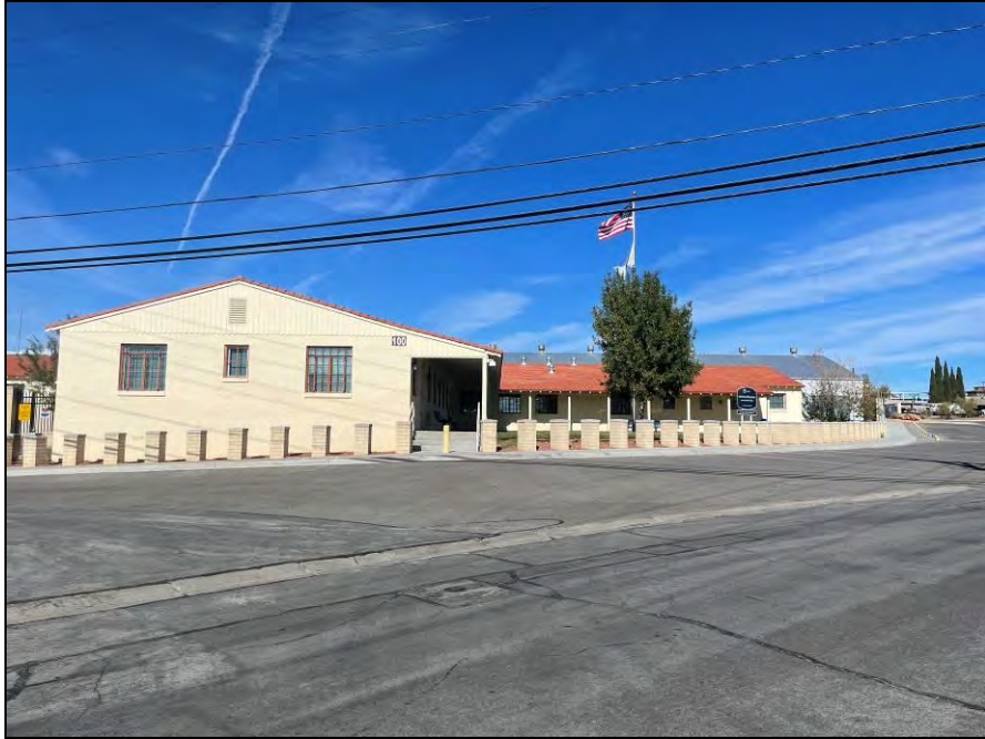
Photograph 5. View of southeast façade of the Training Center and court, facing northwest.
