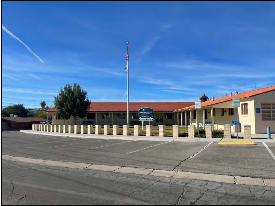
Photograph 7. View of Training Center and court, facing southwest.
