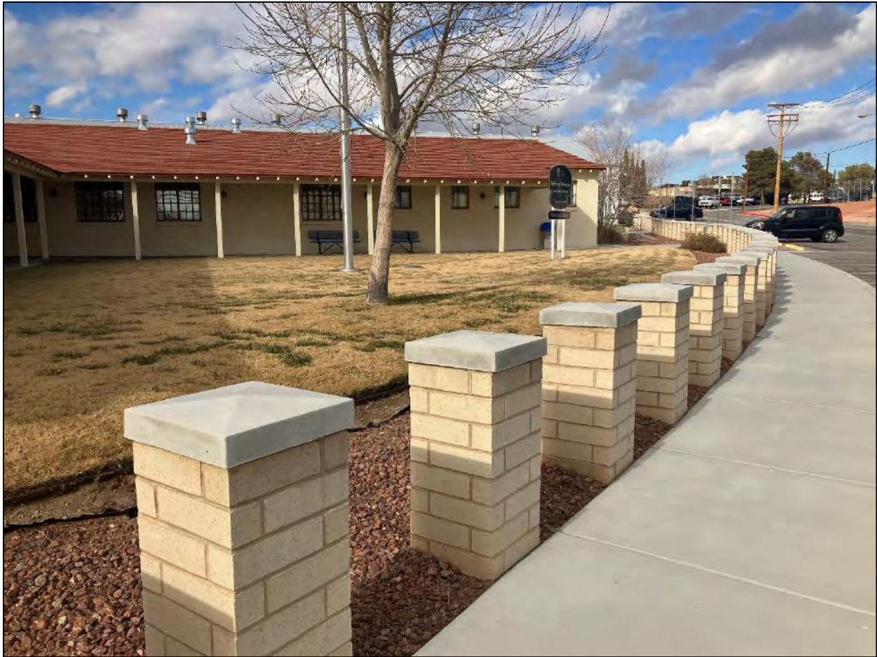
Figure 6. View of southeast façade of the Training Center and court, facing northwest.
