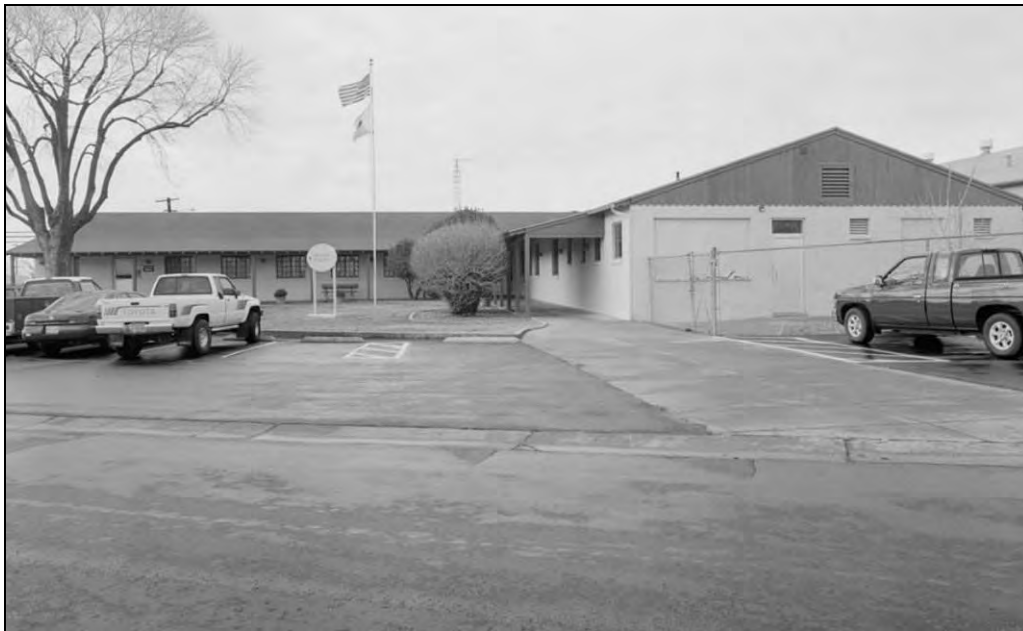
Figure 2. Photograph of landscaped area at the Reclamation Training Center, ca. 1990s (Image courtesy of Historic American Buildings Survey [HABS], Library of Congress, Call No. HABS NV-35-A).
