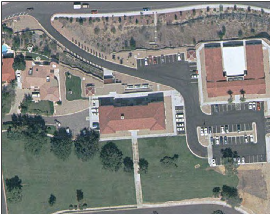
Figure 6. Aerial photograph showing the landscaping surrounding the Administration Building as it appeared in 1998 (Image courtesy of the Clark County Assessor, Las Vegas).
